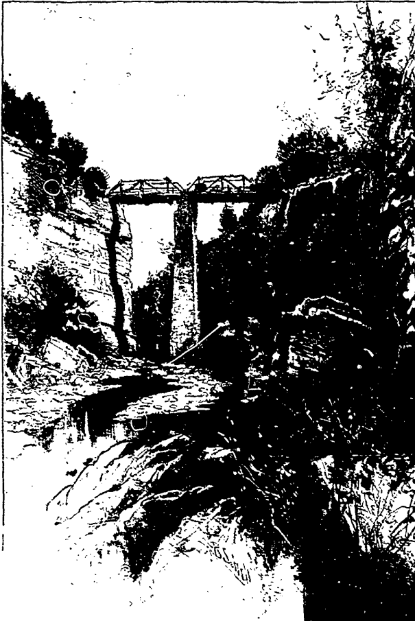
THE BRIDGE, IRVINE RIVER, ELORA.
