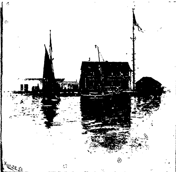
CLUB HOUSE, ST. CLAIR FLATS.
