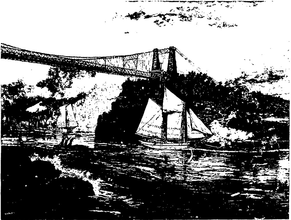
SUSPENSION-BRIDGE, ST. JOHN, AT LOW TIDE.
