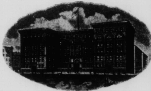
THE MONTREAL OFFICES OF THE MACLEAN PUBLISHING CO. ARE IN THIS BUILDING.
