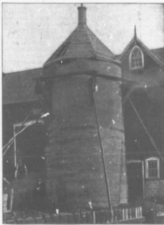
A CEMENT SILO 16 FT. X 35 FT.
