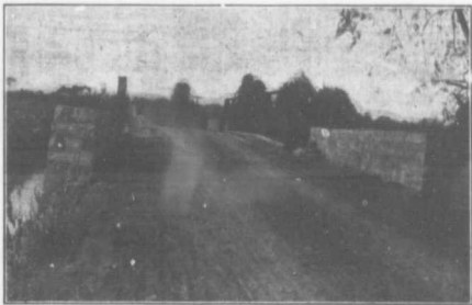
Brandon's Bridge on Lennox and Addington County road system—steel with stone abutments.
