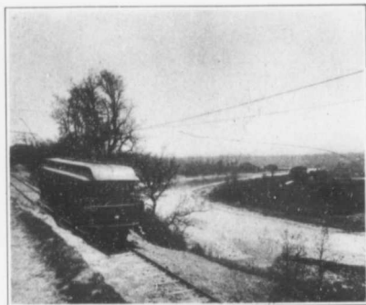
Looking down the River from the Paris Hill.
