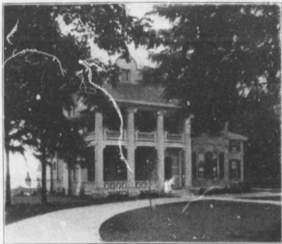
Front View, looking on to Brant Avenue.
