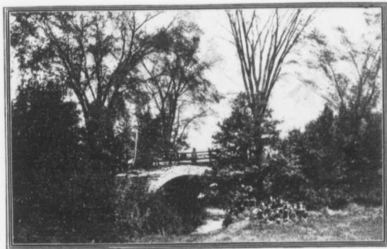
A Historic Bridge in Jackson Park, Galt.
