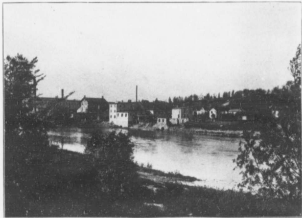
The Rear of The Alabastine Company's Works at Paris, Canada, from the West Bank of the Grand River.
