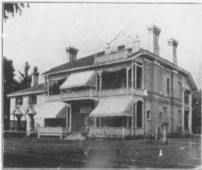
Rear View, overlooking Tennis Lawn, Wooded Hillside and Grand River.
