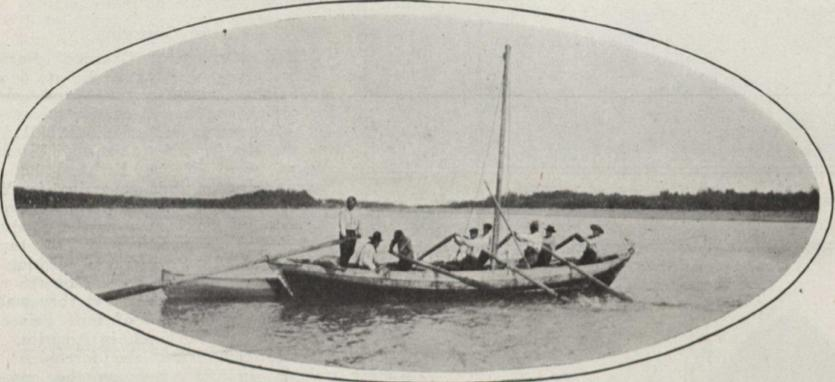
The chief transport of the northern rivers is the York Boat. It is propelled by six sweeps and directed by a seventh. When the wind and current are favourable, a mainsail is used.
