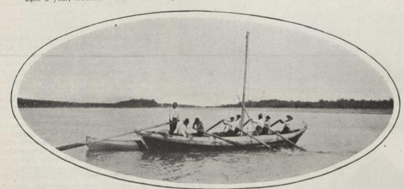
The chief transport of the northern rivers is the York Boat. It is propelled by six sweeps and directed by a seventh. When the wind and current are favourable, a mainsail is used.
