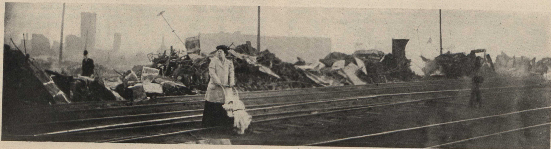
Ruins of Valuable Railway Equipment—View from the Station Platform
