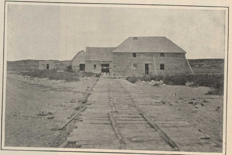
Hudson Bay Company's Whaling Station, east side of Churchill River. Wooden Track put down once a year to bring in Freight from Ship.
