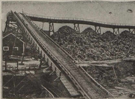
Sometimes the barked or rossed blocks must be conveyed from a rossing plant to the storage yard. Water is the cheapest conveyor, and this picture shows blocks that have been brought by water and are being hauled out and carried by a cable conveyor over a tall tressle, from which they can be dropped wherever desired upon the block pile.
