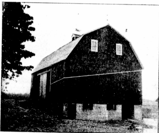
BARN OF WM. PATTON, SOUTH CAYUGA, ONT. Size of basement walls, 31 x 60 x 9 feet. Built with Thorold Cement.
