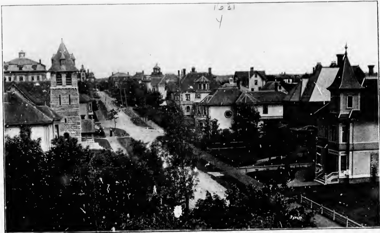
PART OF COLLINS STREET, YARMOUTH.
