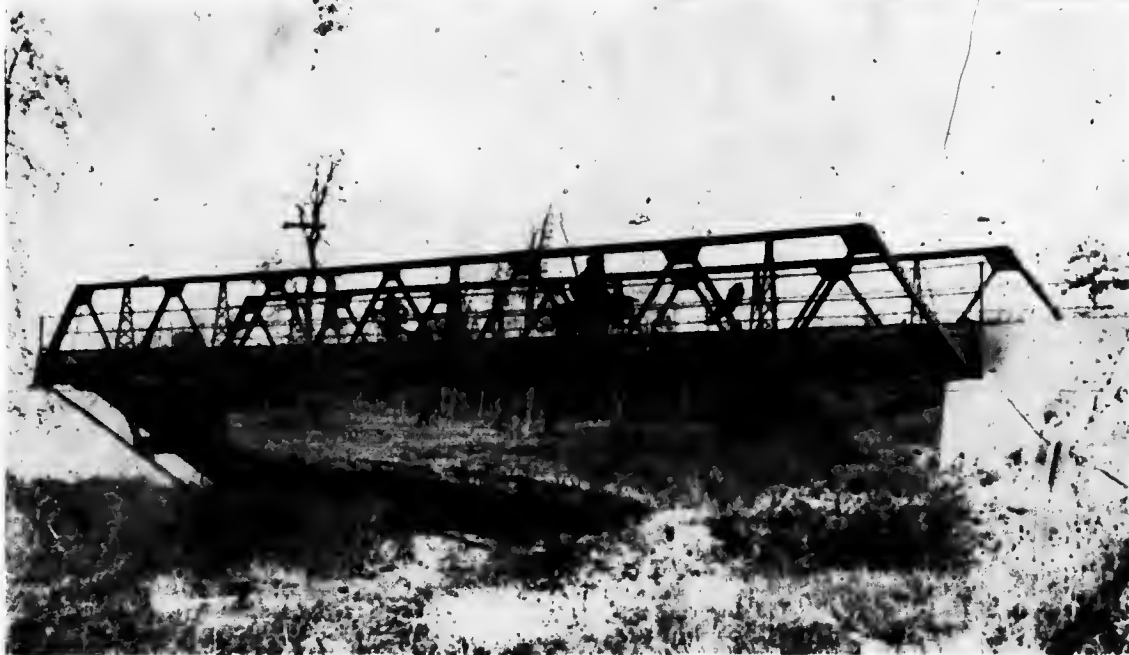
The above is an illustration of steel Warren Truss, span 100' long, erected by us in the Town of Petrolia three years ago. This is a good illustration of another long span Highway bridge built as a low truss. In this case, it was desired to have a low truss to permit the moving and handling of oil derricks without interference with overhead bracing.
