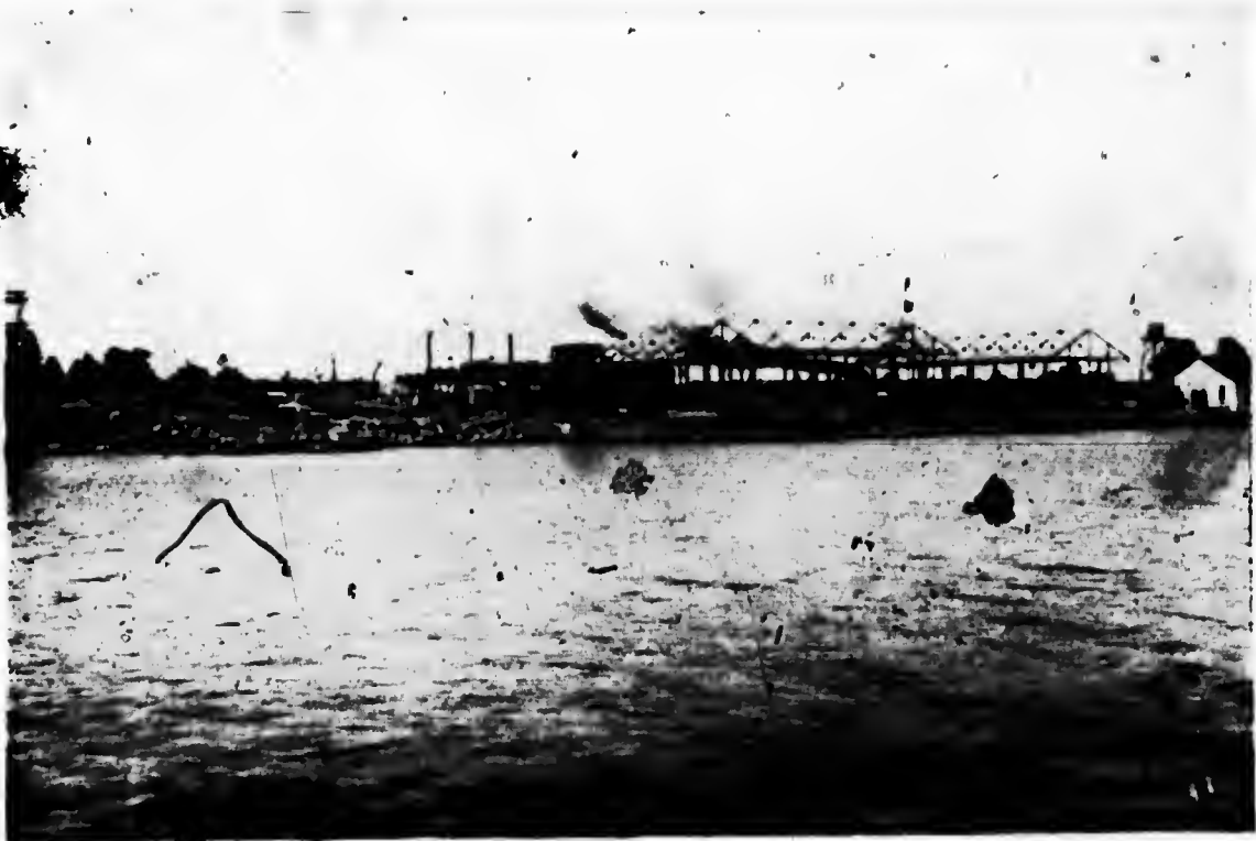
The above cut is a bird's eye view of steel buildings, erected by us, for the Belleville Portland Cement Company, at Point Ann, Ont., near Belleville. Since this cut was made we have erected several additional buildings for this plant.
