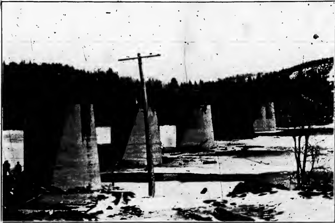
The above illustration represents a bridge on the line of the Canadian Pacific Railway at Aroostook Junction, N. B. This was a case in which our contract covered the removal of four through plate girder steel spans and replacing three of them with deck plate girder spans and the removal of the fourth to the far end of the bridge, and also putting in several additional girders.
