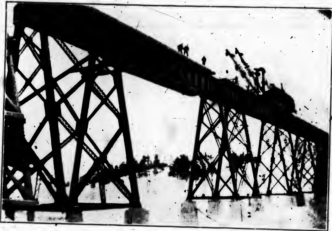
The above photo shows a large portion of Green's Creek Viaduct on the Canadian Northern Ontario Railway, about six miles from Ottawa, Ont., which work was completed by us during the months of January and February, 1909. This work consists of five deck plate girders each 30' long, three deck plate girders each 60' long, and one 80' deck plate girder, all resting on five steel towers each about 50' high. All this work erected with steel derrick car No. 6, no falsework whatever being used.
