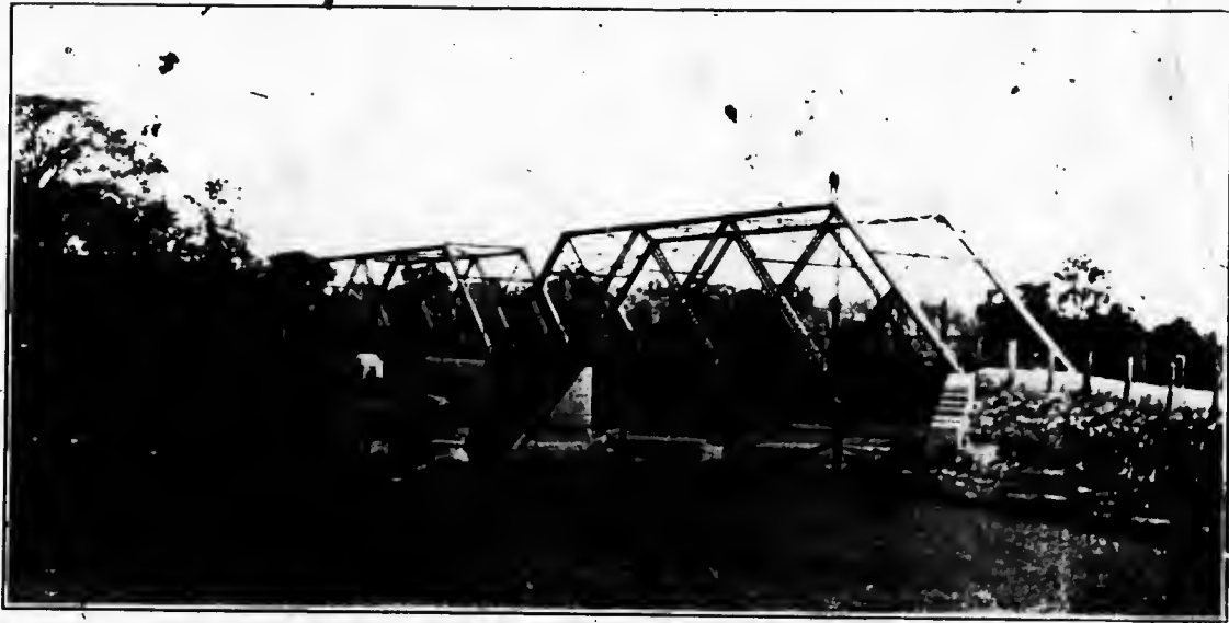
The illustration shows two 150' riveted lattice spans erected by us some time ago for the Township of Woolwich, in the County of Waterloo, and is a good illustration of a first-class highway bridge with concrete floor.
