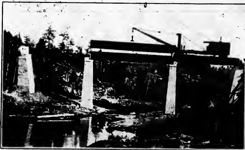
The above is an illustration of one of the several bridges built by us on the Toronto-Sudbury Branch of the Canadian Pacific Railway. The illustration shows our steel erection car placing the second girder of the 90' span.
