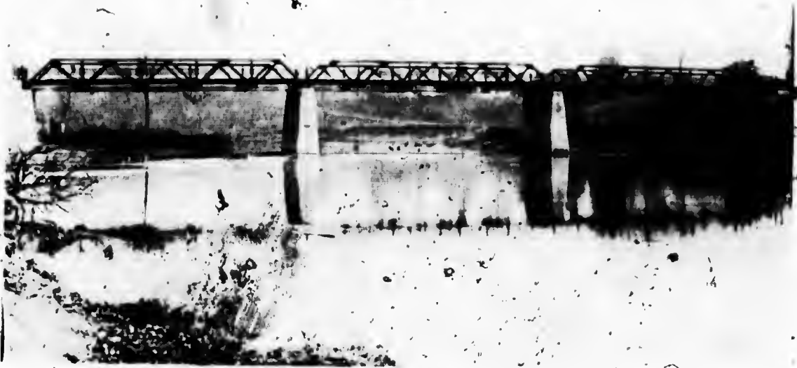
The above illustration shows three Warren Truss Steel Highway Spans, built by us near London, Ont., and known as Plover Mills Bridge.
