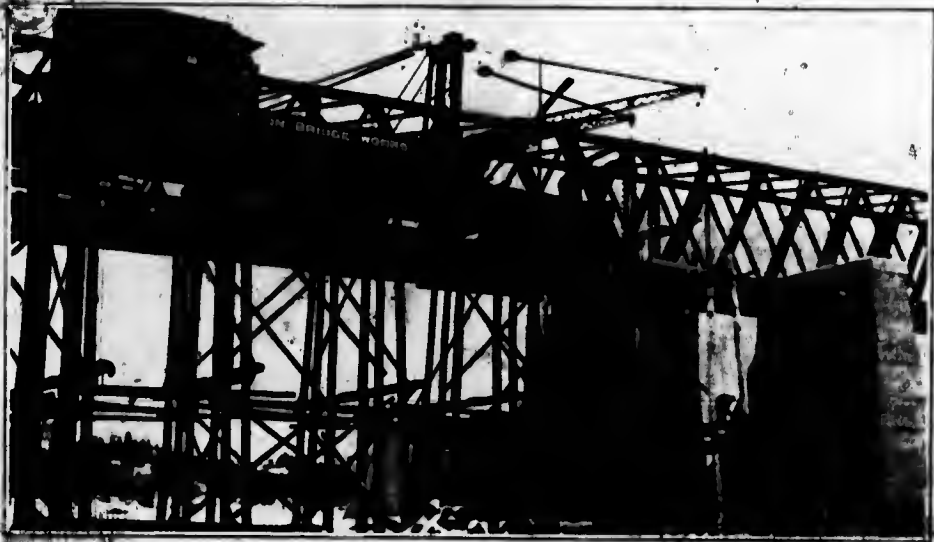
The above photo is another illustration of Canadian Pacific Railway Bridge, at Upper Woodstock, N. B., and shows the method of placing falsework on which to erect the new steel structure. It will be seen that our steel erection car is not only used in placing long and heavy girders but is also adapted for handling timber, etc., in the placing and building of falsework.
