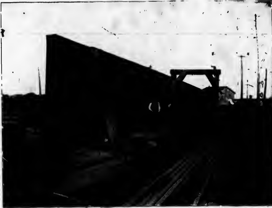
Centre Girder of Street Subway, Toronto, on the line of the Grand Trunk Railway System. over all; Weight 87,000 lbs.
