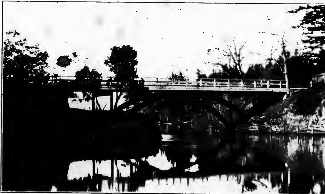
The illustration shows a Steel Arch, erected by us some years ago over Victoria Arm on Vancouver Island.
