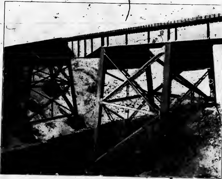
Steel Plate Girder Double Track Skew Crossing over Desjardins Canal, Hamilton, on the Toronto, Hamilton & Buffalo Railway. Length over all, 219'; weight 475,000 pounds.
