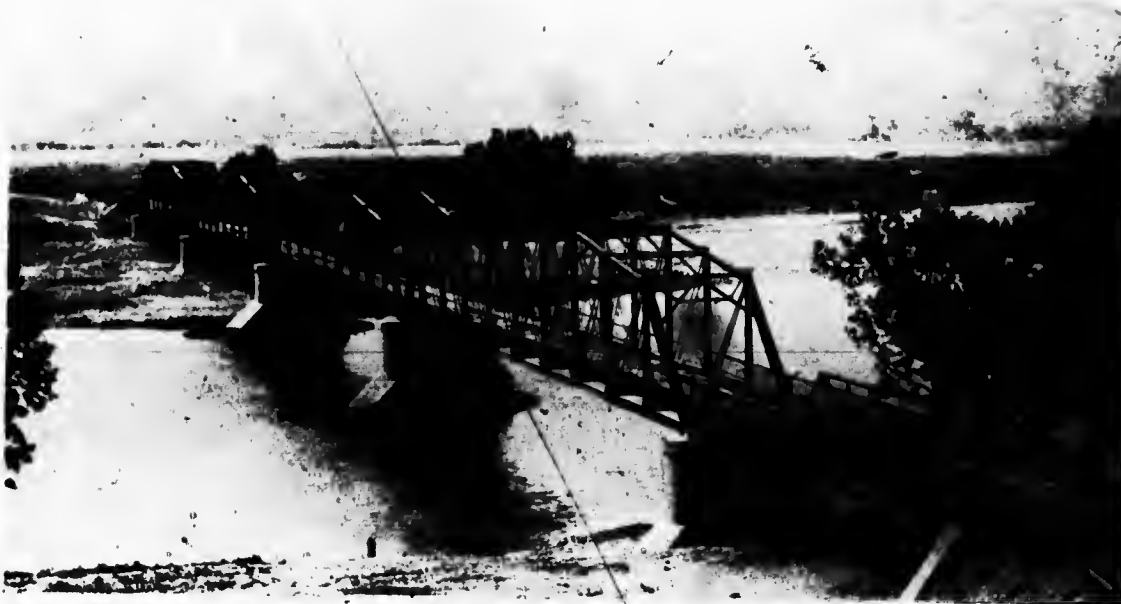
The above illustration shows the steel bridge built by us several years ago for the Government of the North-West Territories, and is over the Belly River at Lethbridge. It consists of four 175' Pin Connected Spans, and two 80' Riveted Warren Truss spans all with a 16' roadway. On page No. 12 will be found an illustration, showing the very handsome concrete piers used for this bridge.
