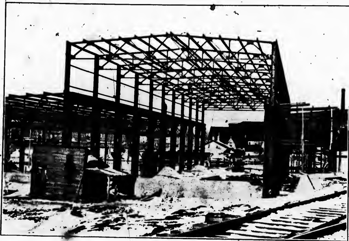
The above cut illustrates the structural steel erected by us in the new Foundry Building for the McGregor, Gourlay Company, of Galt, in 1906. This illustrates the latest type of construction used in buildings for foundry purposes. It will be noted the steel trusses are supported on steel columns and that there are steel runways to support heavy travelling crane.
