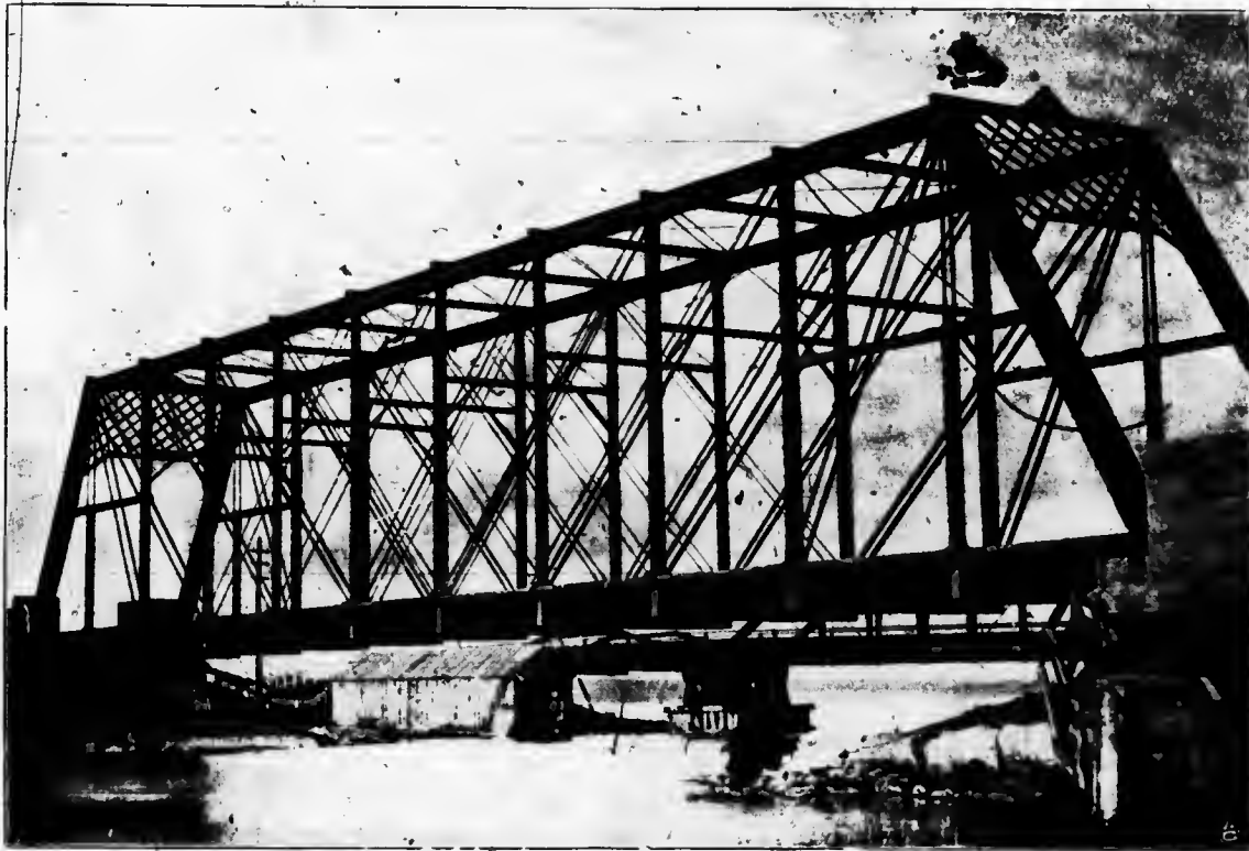
Single Track Through Pin Connected Span, carrying the line of the Grand Trunk Railway over the Humber River. Span, 202'; weight 450,000.
