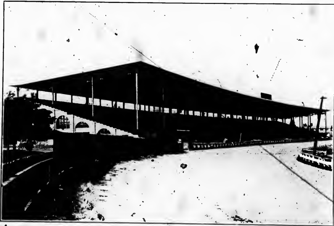
The above cut illustrates a view of the Grand Stand at Toronto Exhibition Grounds fully completed, with concrete terrace, roof, etc., etc.
