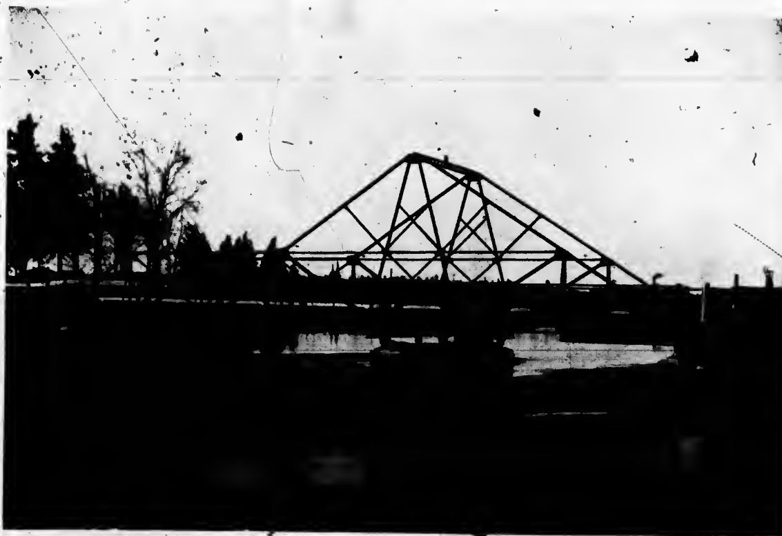
This cut illustrates a light highway swing bridge erected by us at Kemptville, some years ago, and is one of several similar spans erected in different parts of the country.
