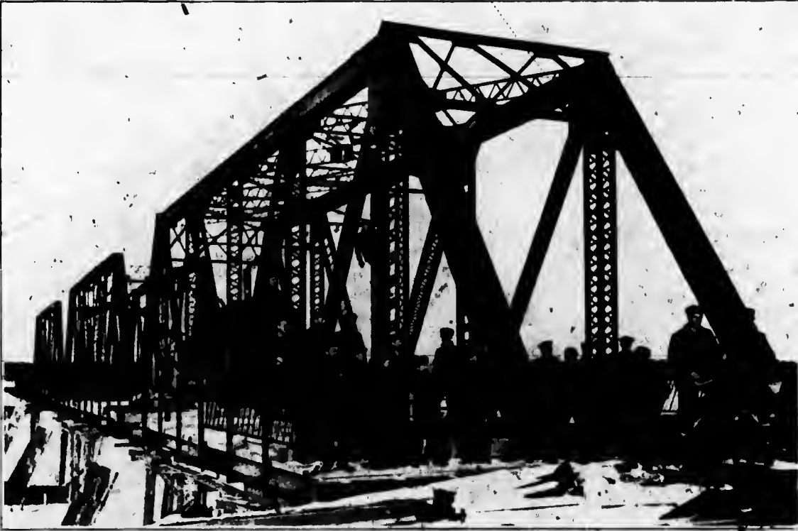
Canadian Northern Railway Bridge, Prince Albert, Sask.
