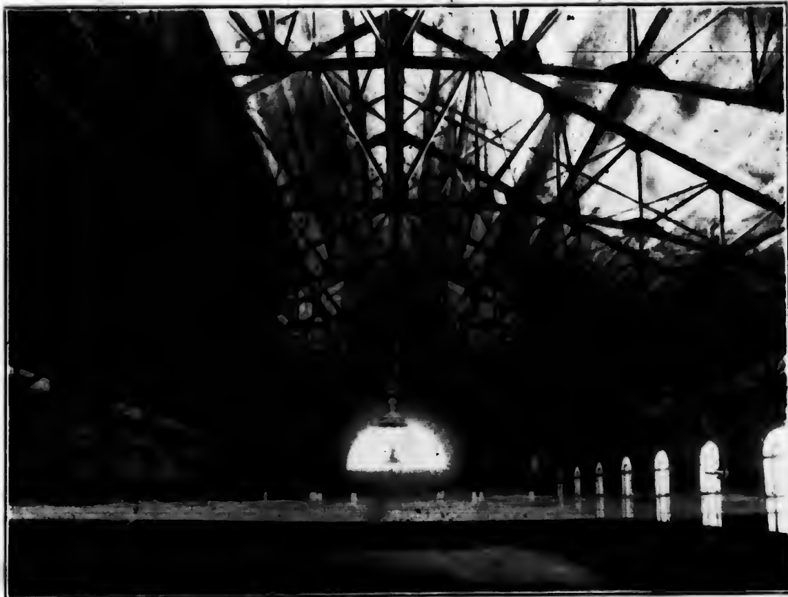
The above illustration shows steel roof on new Drill Hall and Armories recently erected in the City of Hamilton. This steel is heavy and pleasing in outline. The span of the roof is 130' face to face of walls with a total length of 240' and the height from the under side of the bottom chord at the centre of the truss to the floor of the hall is 52' feet. The netting shown at the bottom of this illustration is placed to permit the playing of indoor baseball and which is necessary to protect the electric lamps and windows.
