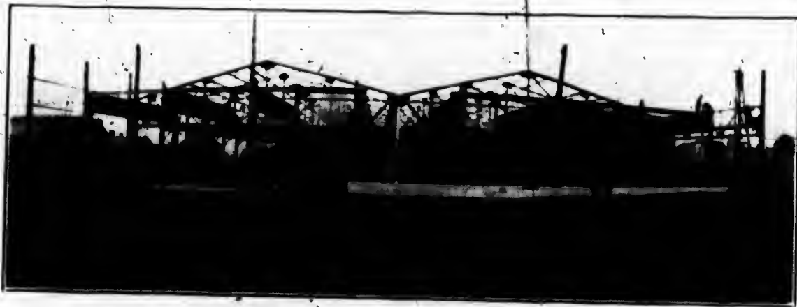
This illustration shows the steel work of our new bridge shops in the course of erection and nearly completed, and ready to receive the roofing and siding.
