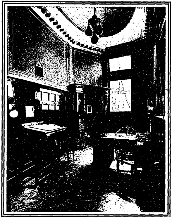
MANAGER'S OFFICE, BANK OF BRITISH NORTH AMERICA, WEST TORONTO. ELLIS & CONNERY, ARCHITECTS.
