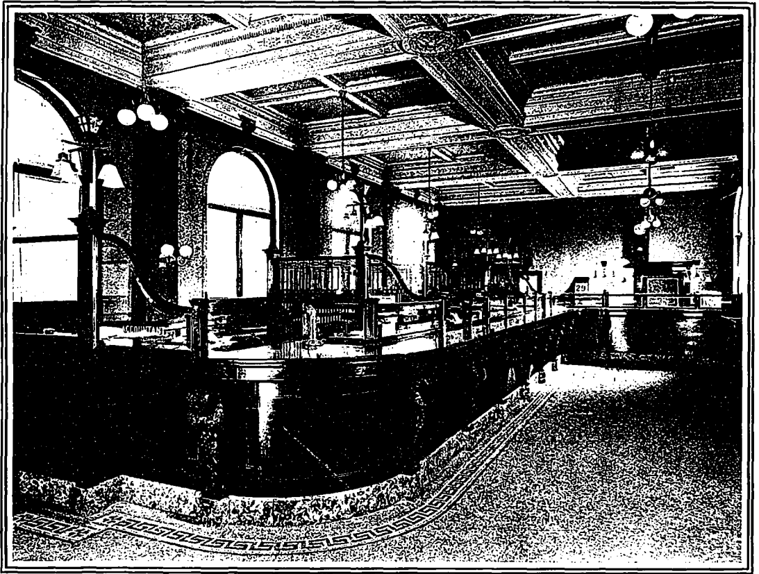
MAIN BANKING ROOM, SHOWING A DEVIATION FROM CONVENTIONAL HEAVY GRATING AND GRILL WORK IN BANK FIXTURES, BANK OF BRITISH NORTH AMERICA, WEST TORONTO. ELLIS & CONNERY, ARCHITECTS.
