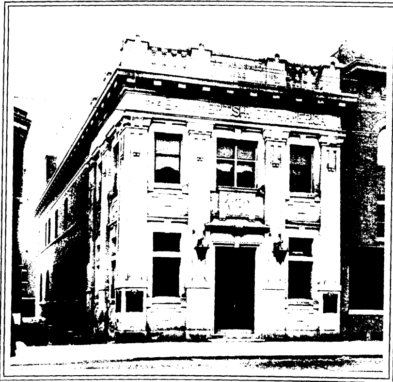
Bank of British North America, Toronto Junction — Ellis & Convery, Architects, in which Milton Pressed Brick was used.
