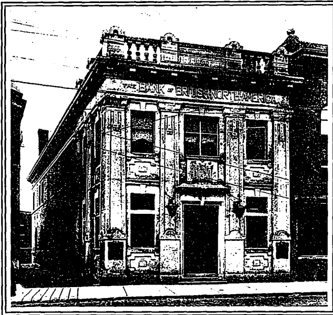
BRANCH BANK BUILDING, BANK OF BRITISH NORTH AMERICA, WEST TORONTO ELLIS & CONNERY, ARCHITECTS.
