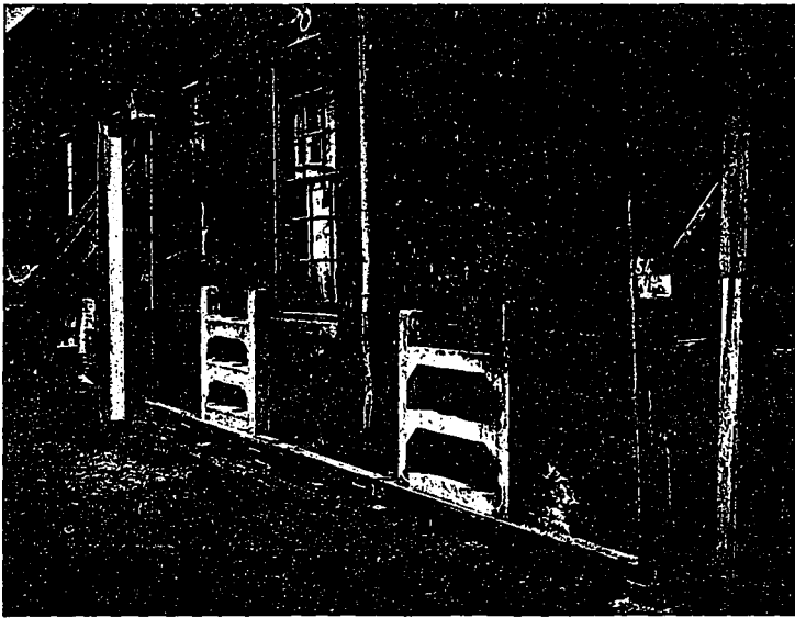
PLATE NO. 2—EXPERIMENTS TO DETERMINE THE FLOW OF CONCRETE IN WOOD FORMS 4 IN. SQUARE IN CROSS SECTIONS.
