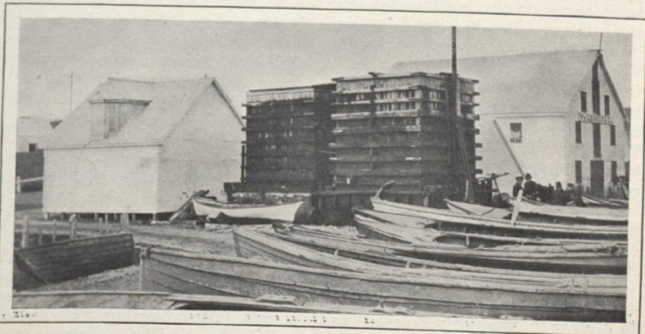
VATS FOR HOLDING SEAL OIL
