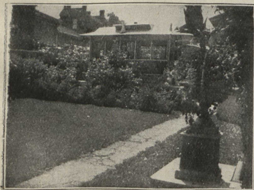
FIG. 2471. A STREET CAR USED AS A SUMMER HOUSE, MAIN ST., HAMILTON.
