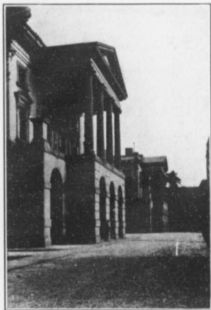
South Facade Osgoode Hall
