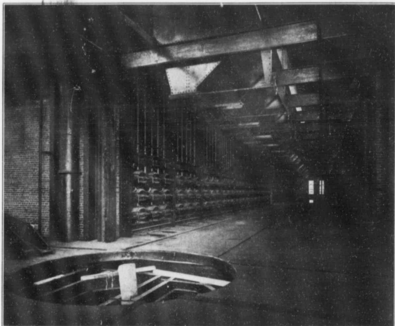
End of Retort House the Consumers' Gas Company (Daily capacity 5,000,000 cubic feet)
