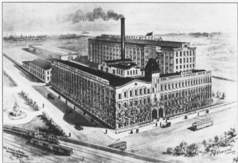
Head Office of The Toronto Carpet Company, Limited
