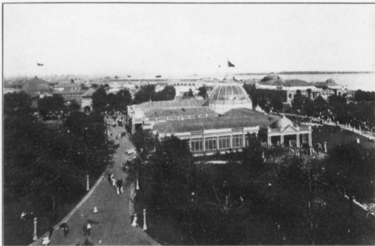
View looking east, taken from the Transportation Building
