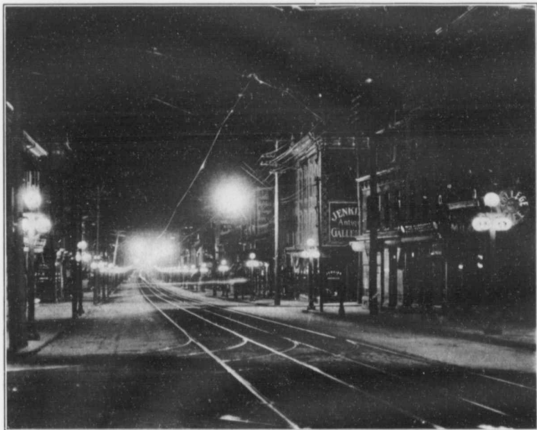
A Business Street showing the Cluster Lights of The Toronto Hydro-Electric System
