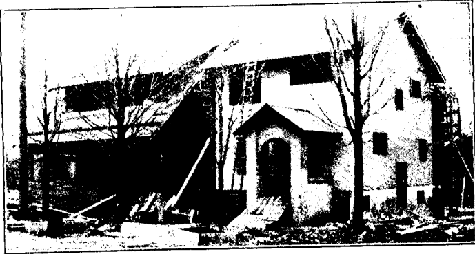
Houses erected by B. A. Grison, Esq., Ottawa, Ont. Outside walls of 2 x 4 studding. Stucco Board on exterior. Sheathing Board on interior. Over Sheathing Board, a 1 x 2 Furring was applied, then Stucco Board and Plaster, giving double air space, increasing the warmth, yet keeping down the cost.
