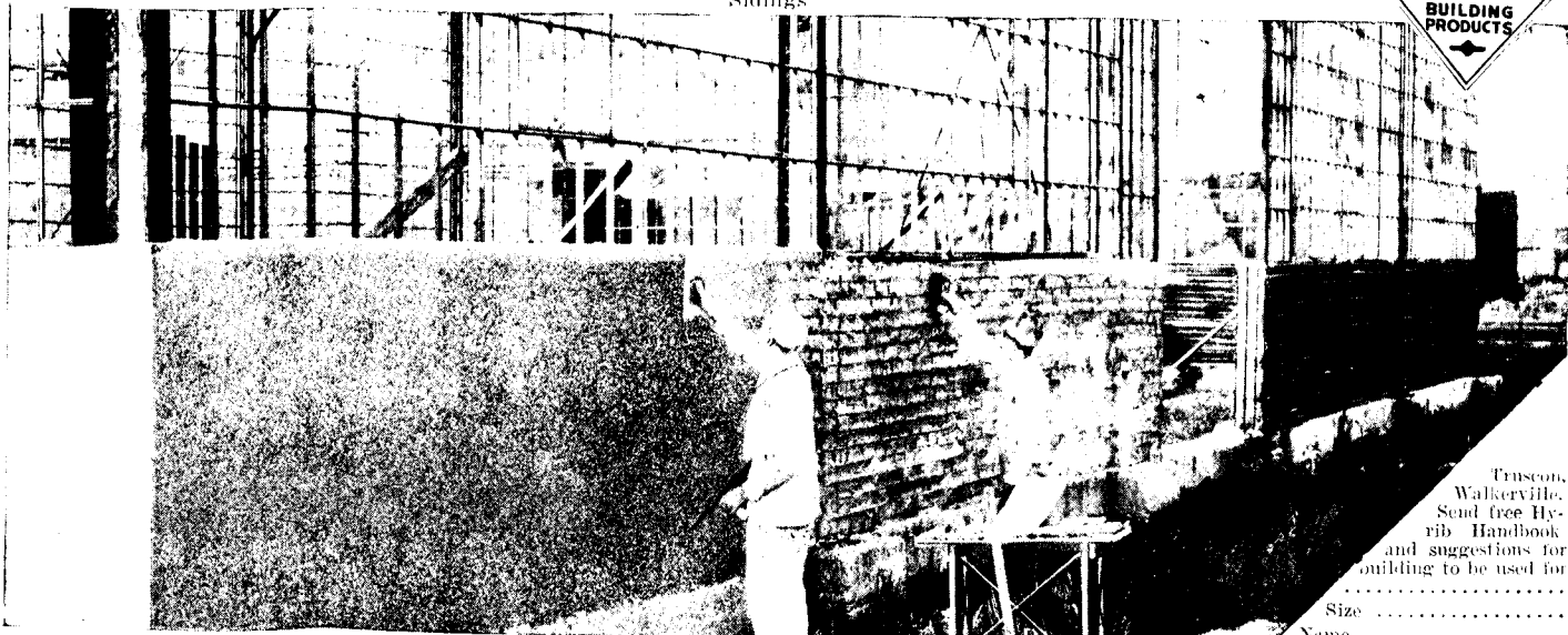
Plastering Hyrib Sidings
