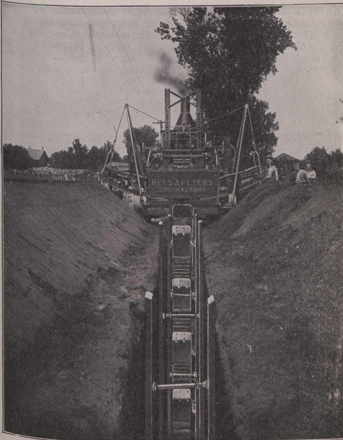
Parsons Excavator-Carlsbad, N.M.
