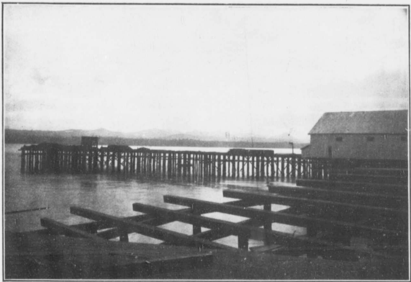
Whaling Station at Naden Harbor during Construction
