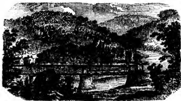
VIEW OF THE IRON BRIDGE AND SCENERY AT ELLYSVILLE, TWENTY-ONE MILES FROM BALTIMORE.
