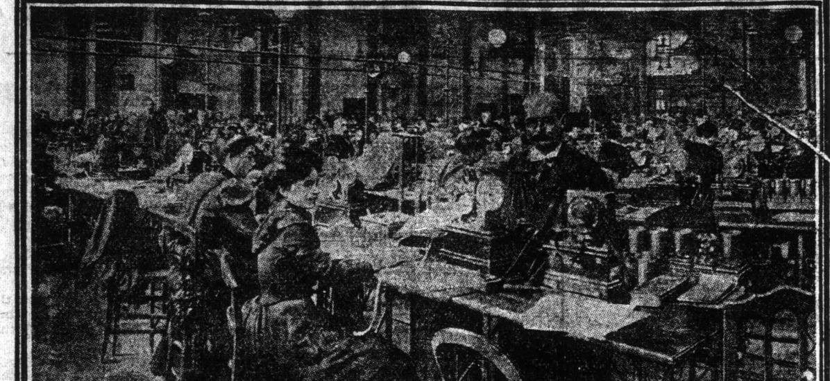
MAIN OPERATING ROOM OF THE PARIS CENTRAL TELEPHONE EXCHANGE.
