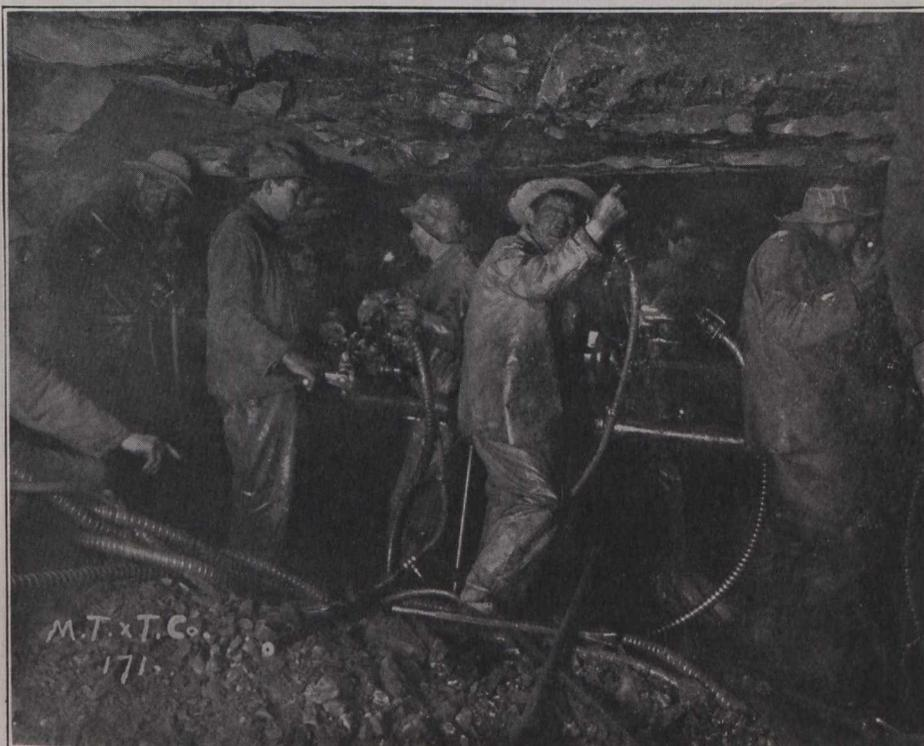
Mount Royal Tunnel—Heading. Observe Drills on Horizontal Bar and Water Attachment to Drills.
