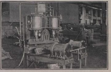
Air Press for Straightening Brake Beams.
