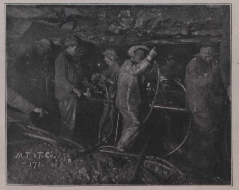
Mount Royal Tunnel-Heading. Observe Drills on Horizontal Bar and Water Attachment to Drills.
