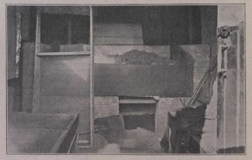
Electrically Heated Sand Drying Plant.
