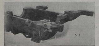
Motor Cases Can Be Welded With Thermit in a Few Hours, and Kept Them From the Scrap Heap.
