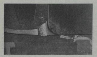
Sternshoe of a Vessel Welded With Thermit, and the Vessel Was Taken Off the Drydock in Less Than Three Days.
