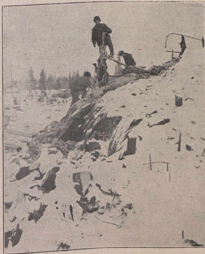
Excavating for Mill at the Dome.
