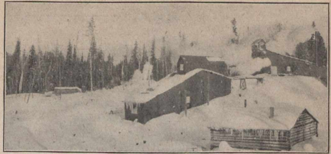
Mill and Power Plant at Vipond
