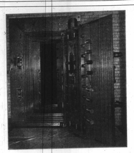
Vault doors in Bank of Montreal and Royal Trust Company, Montreal Three times larger and heavier than any other in Canada. Doors and Vestibules weigh 60 tons. Total weight of lining and doors 260 tons. bules weigh 60 tons. Total weight of lining and doors 260 tons. Accepted to be the finest piece of vault work in construction and workmanship in the Dominion. — Built by the old established firm of
