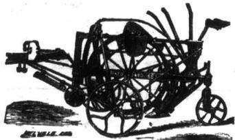
**ELEVATOR DITCHING MACHINE FOR UNDERDRAINING.**
