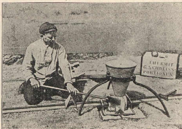
Railwelding by means of Thermit.
