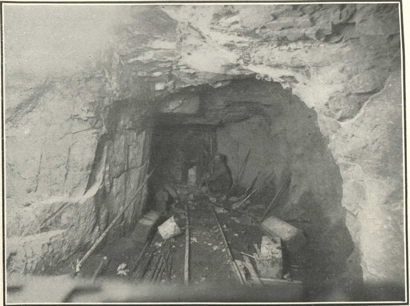
A Tunnel in a Silver Mine at Cobalt.
