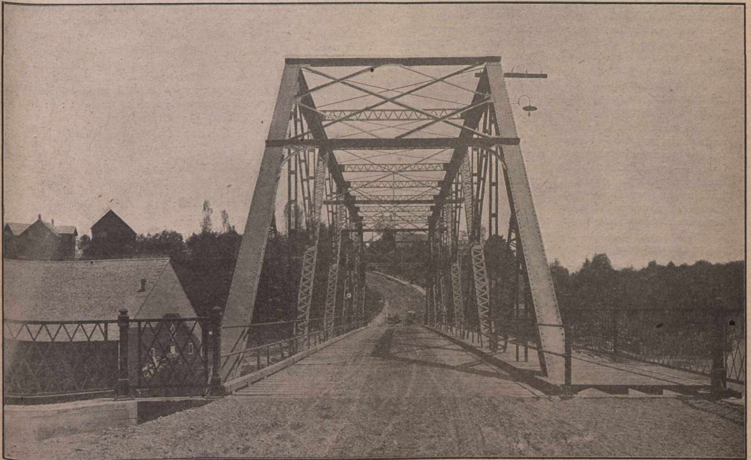
BRIDGE ACROSS MUSKOKA RIVER, THOMAS STREET, BRACEBRIDGE
