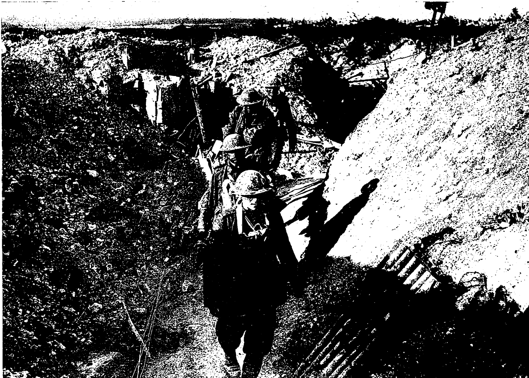
Daylight "clearing" through a Trench.
