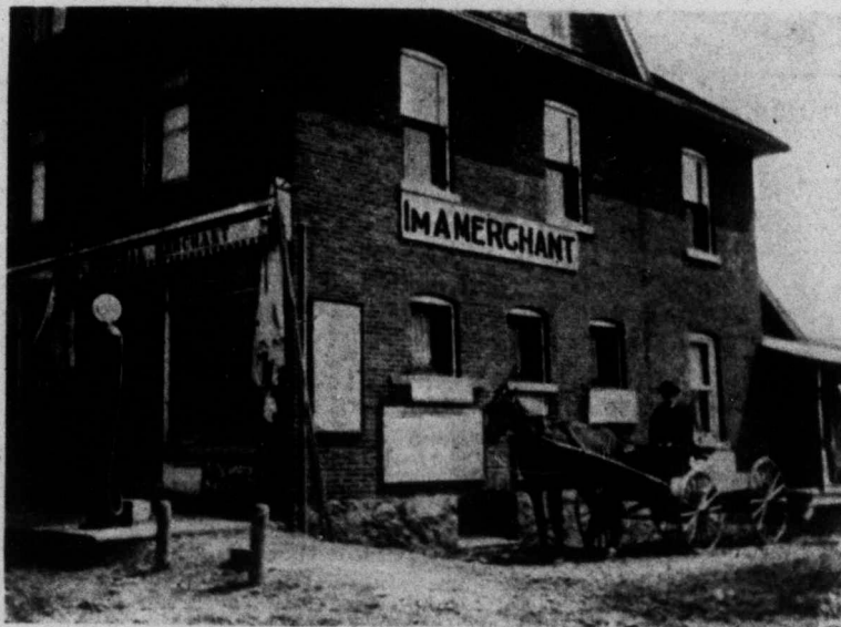
A view of the store of A. Kirkpatrick, Lefroy, Ont. Full details are to be found in the accompanying article. Notice the automatic gasoline filling station.
