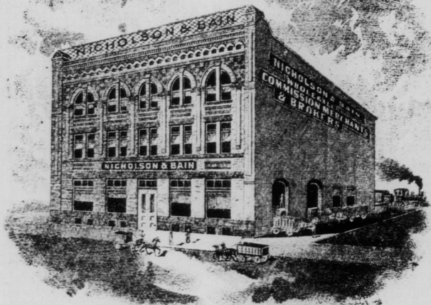
BANNATYNE ST EAST TRANSFER TRACK.
