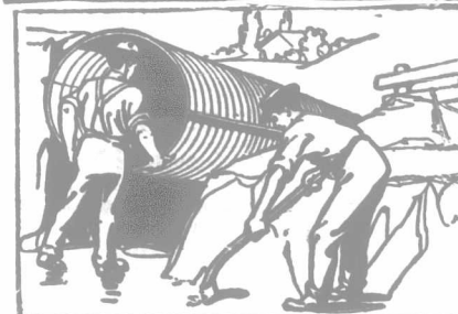
The above two pictures tell the whole story of installing a frost-proof, time-proof Pedlar Nestable Culvert.
