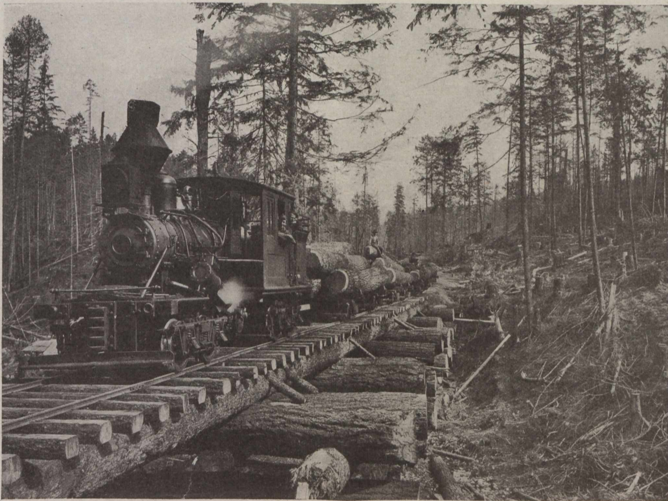
A Logging Railway, showing type of engine used and method of putting down the tracks.
