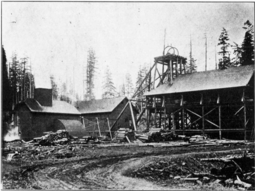
No. 5 Shaft, Looking North, Cumberland.
