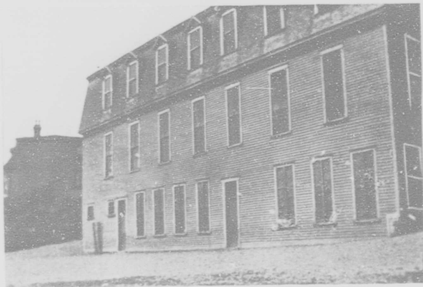
CENTENARY HALL ELEMENTARY SCHOOL
