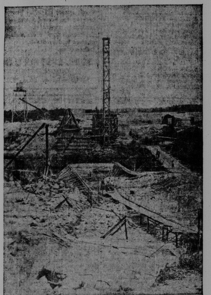
Concrete Pouring Tower at the East Branch Dam.
