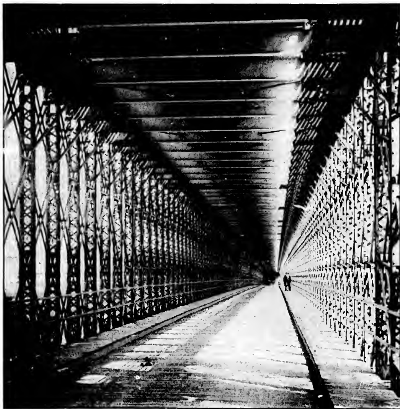
SUSPENSION BRIDGE ROADWAY.
