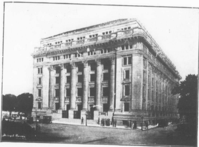
PROPOSED NEW HEAD OFFICE BUILDING OF THE SUN LIFE OF CANADA, DOMINION SQUARE, MONTREAL.
