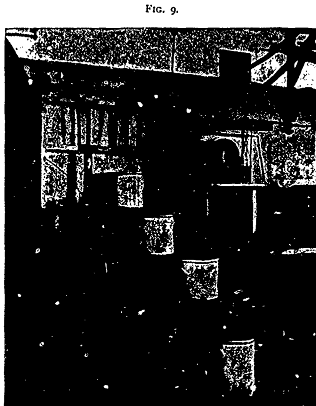
Leaching-Tubs Arranged for Mechanical Stirring.
