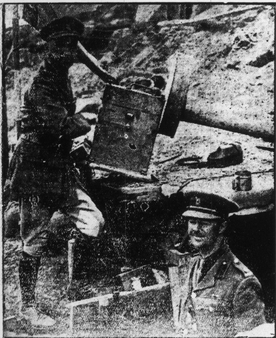
Captain the Hon. W. J. Shaughnessy (On left) taking the bad air from his dug-out with a captured machine made for the purpose.
