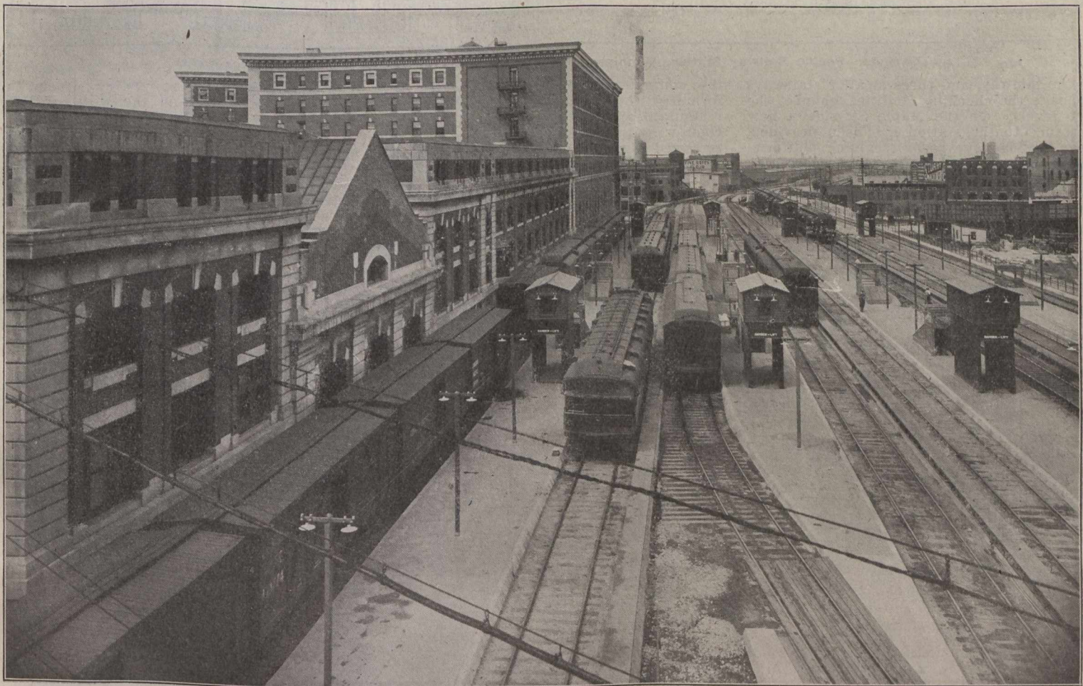
Passenger Tracks and Platforms, Canadian Pacific Railway Station, Winnipeg, Looking West.
