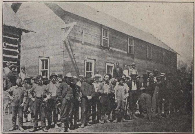
Mining and Construction Crew, Graphite Limited
