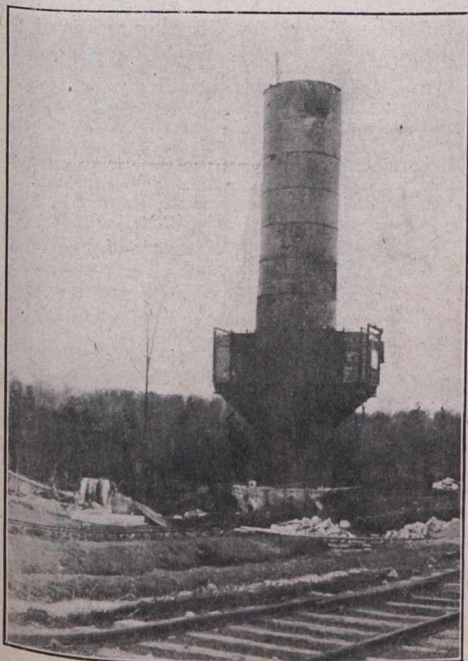
Lime Kiln in process of construction at Missisquoi Marble Quarry
