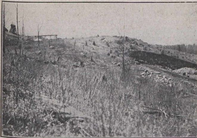
Graphite Limited, Shaft House to left, Mill Site to right
