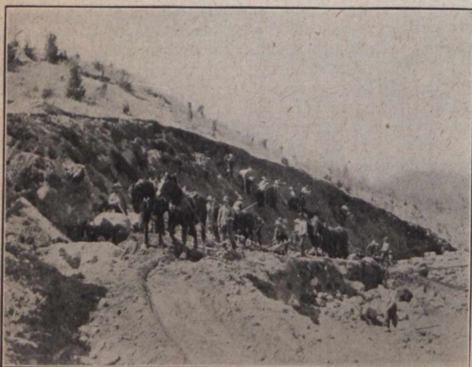
Excavation for Mill, Graphite Limited
