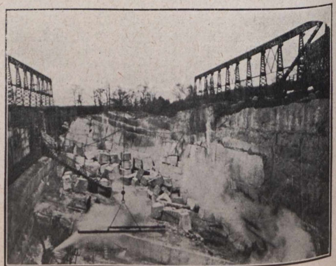
View of Missisquoi Marble Quarry
