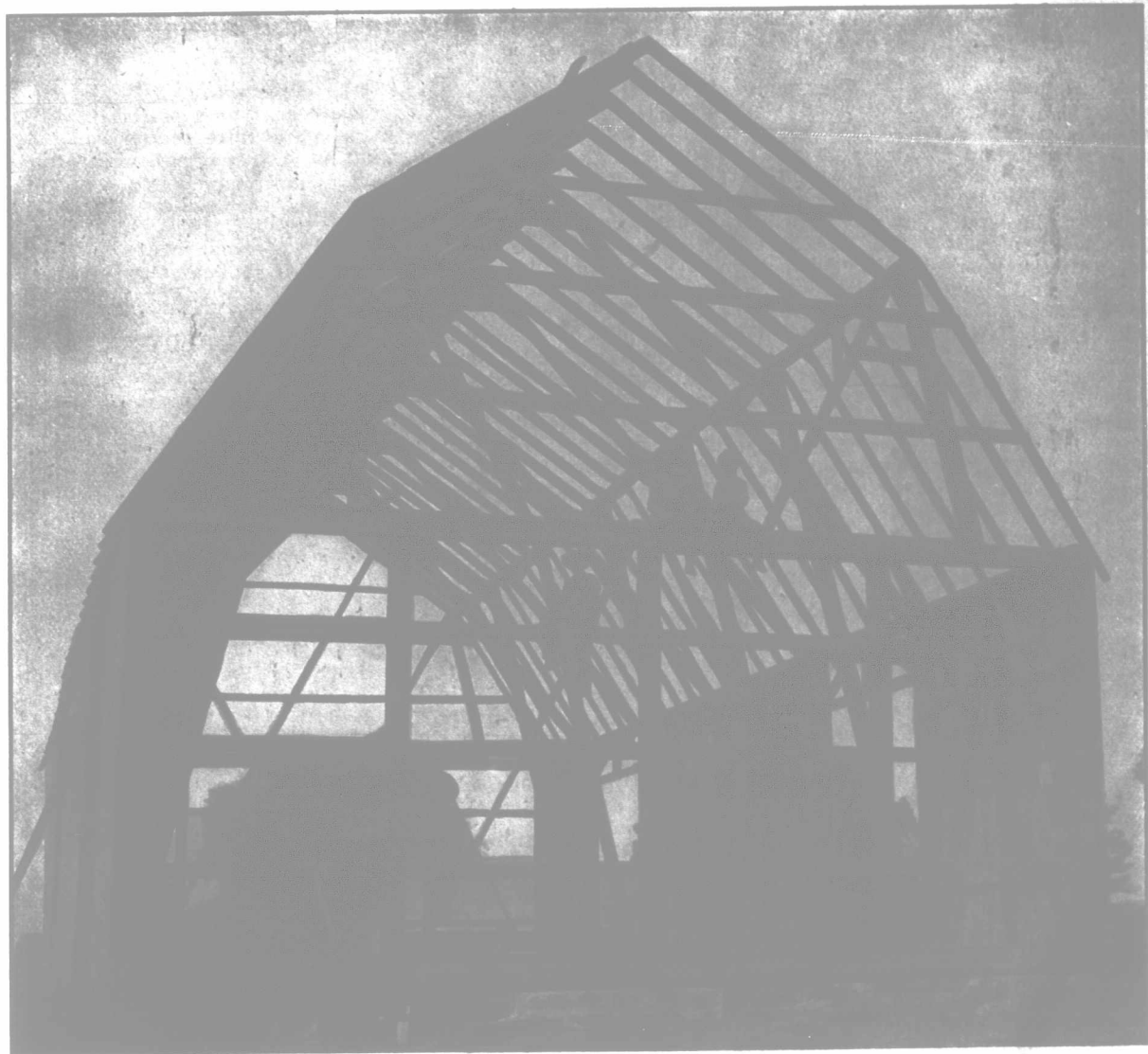
Plank-frame Barn, Built by Alf. A. Gilmore, Huntingdon, Que.
