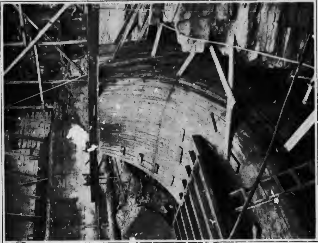
No. 4 draft tube forms in position ready for concreting
