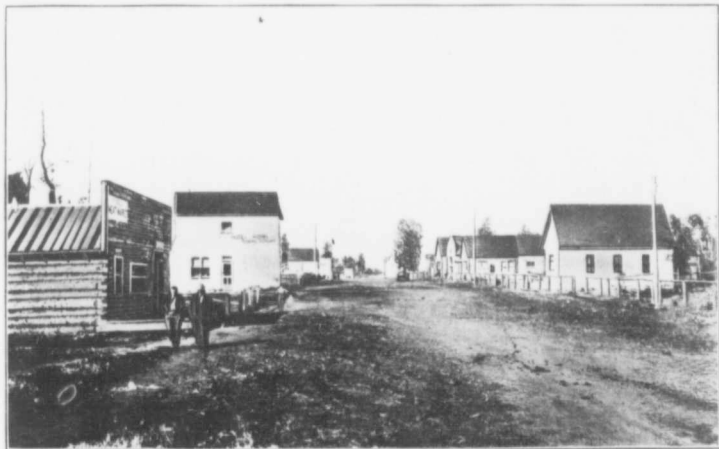
PLATE 13.—Main Street of Gronard, Alta., Looking West.
