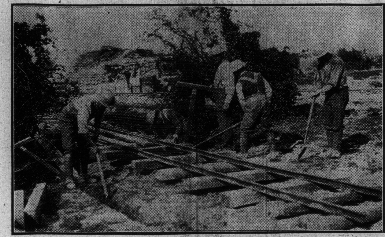
CANADIAN OFFICIAL PHOTOGRAPH FROM THE WESTERN FRONT. Canadian railway troops, working in shelled area, laying track, which will end within a few hundred yards of enemy trenches.
