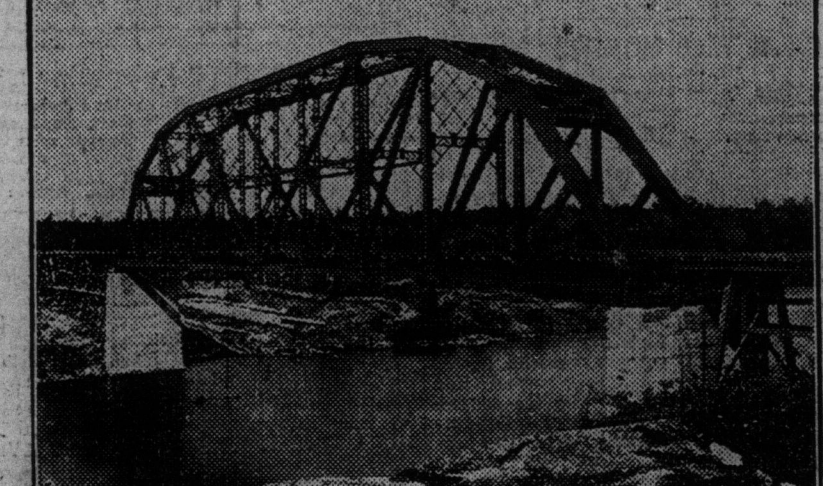
BRIDGE OVER THE PICKEREL RIVER, ON THE C.N.R. LINE TO SUDBURY—SPAN 296 FT.; CENTRE HEIGHT 52 FT.
