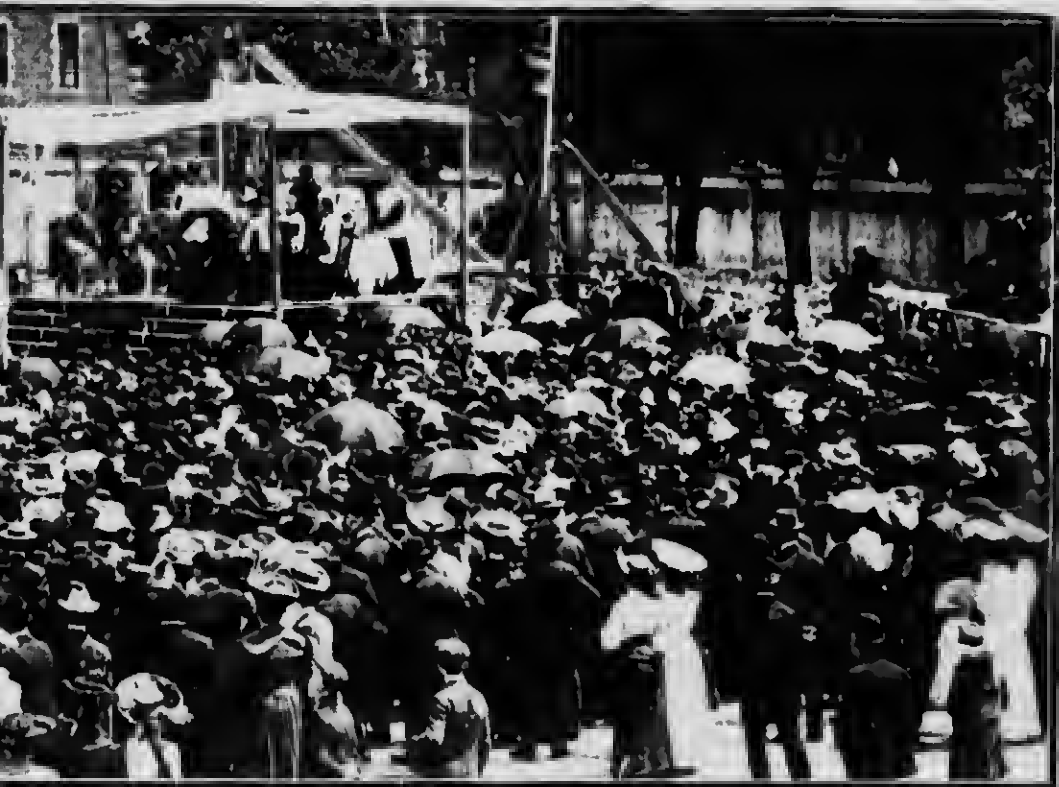
ER ST NE OF THE NEW ARTS BUILDING.
