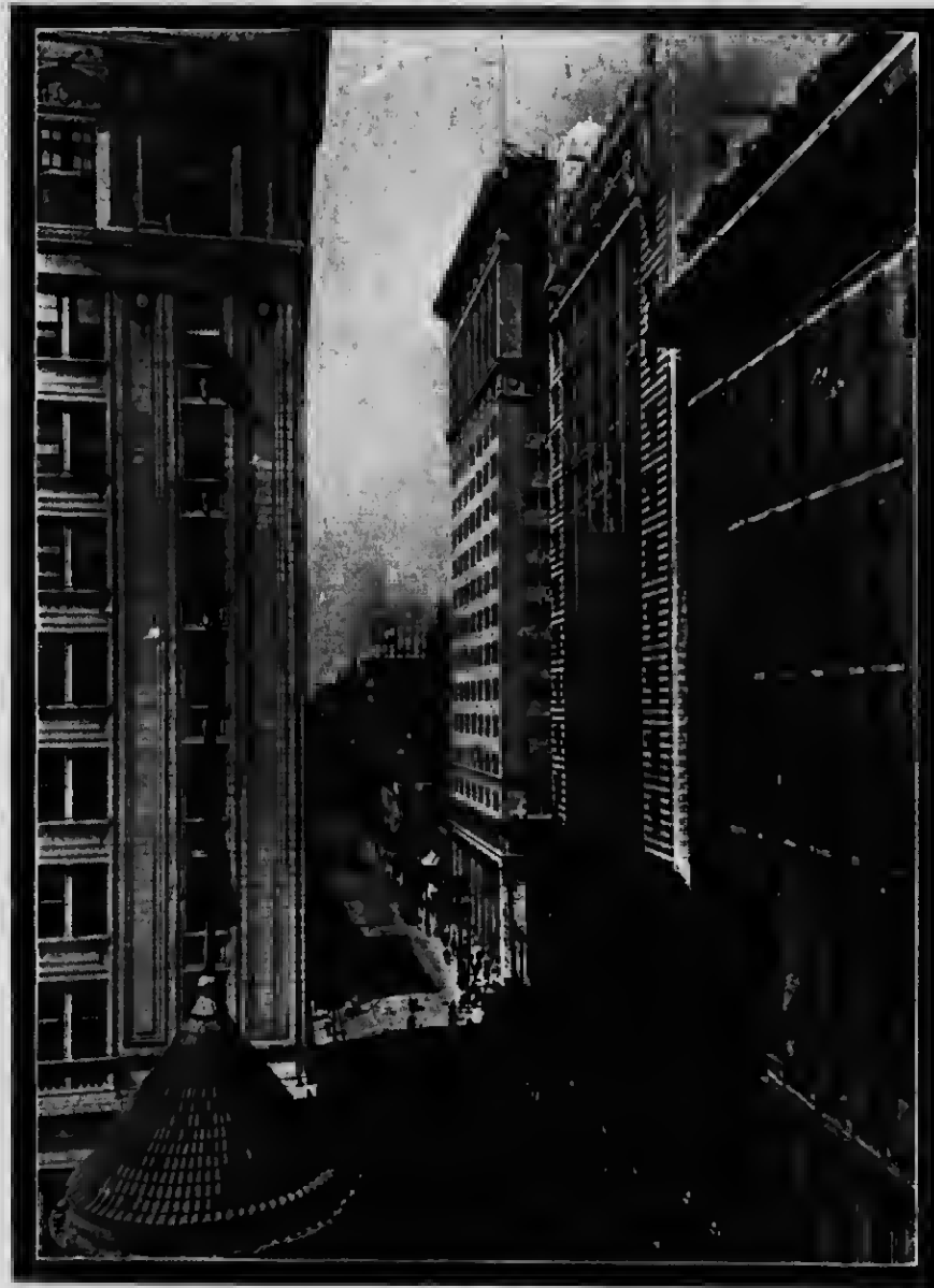
A GROUP OF DOWNTOWN OFFICE BUILDINGS, TORONTO.
