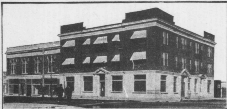
Smith Block and International Hotel, 12th Ave., Estevan
